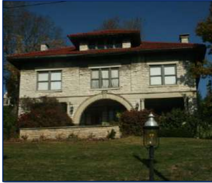
946 Redway Ave. (Elzner & Anderson)
